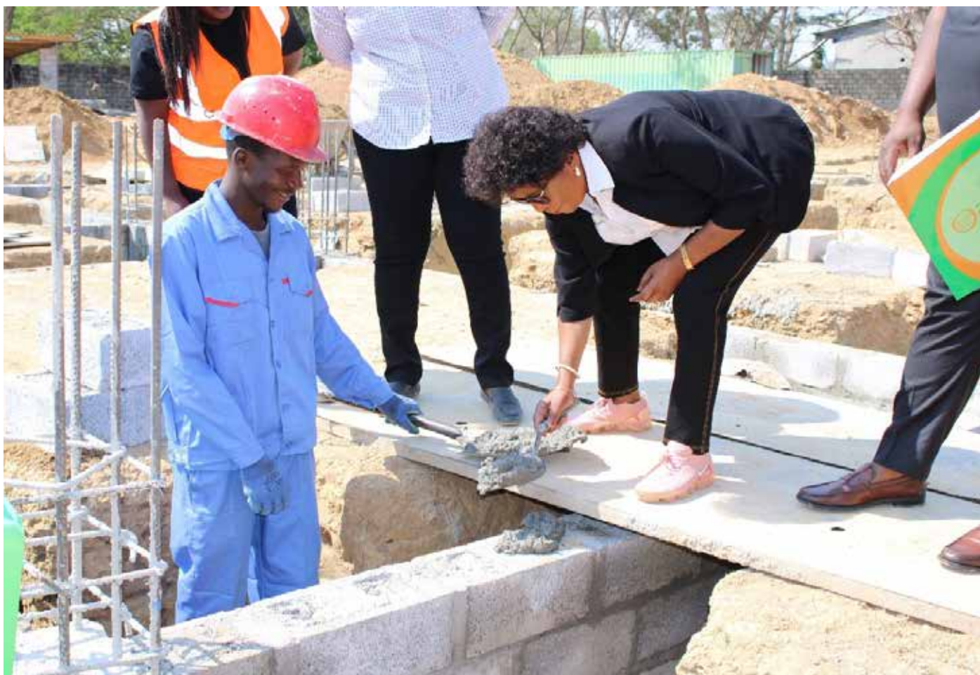
ZPPA DG Mrs. Idah Chella during the commissioning of the annex building project.
